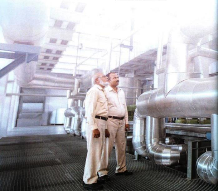
Your Company has also installed an environmentally friendly gas based power plant with a view to reduce power cost. Moreover, it produces steam as a by - product which is adequate to meet the entire steam requirements of Polyester plant of the Company thereby resulting in energy conservation.
