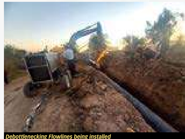
Debottlenecking Flowlines being installed
