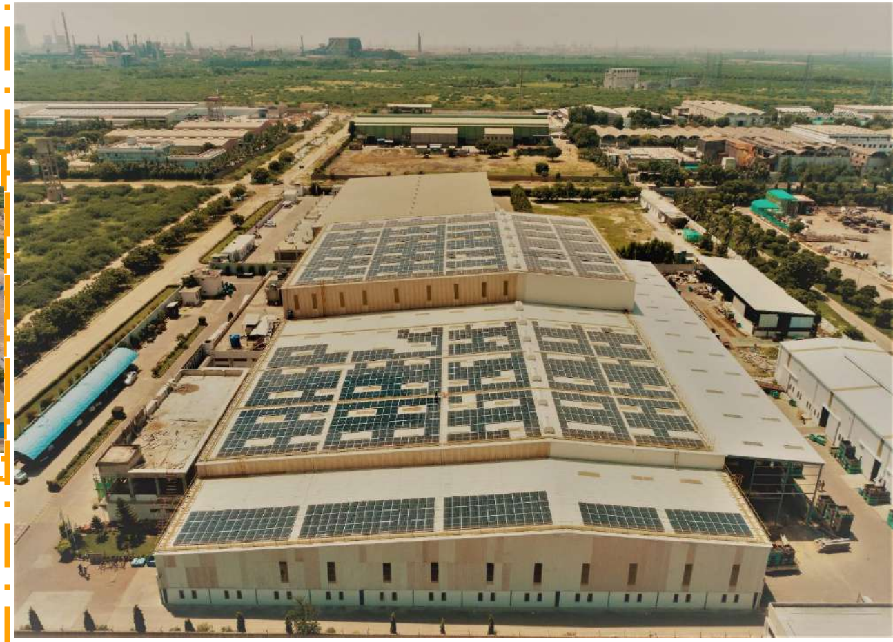
1 MW Solar Plant at ASC
