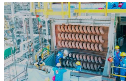
Furnace Steam Coil (KS Coil) Replacement
