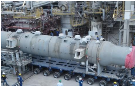
Waste Heat Boiler Replacement
