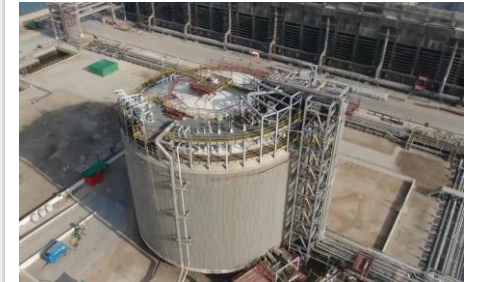
Ammonia Storage Tank Inspection
