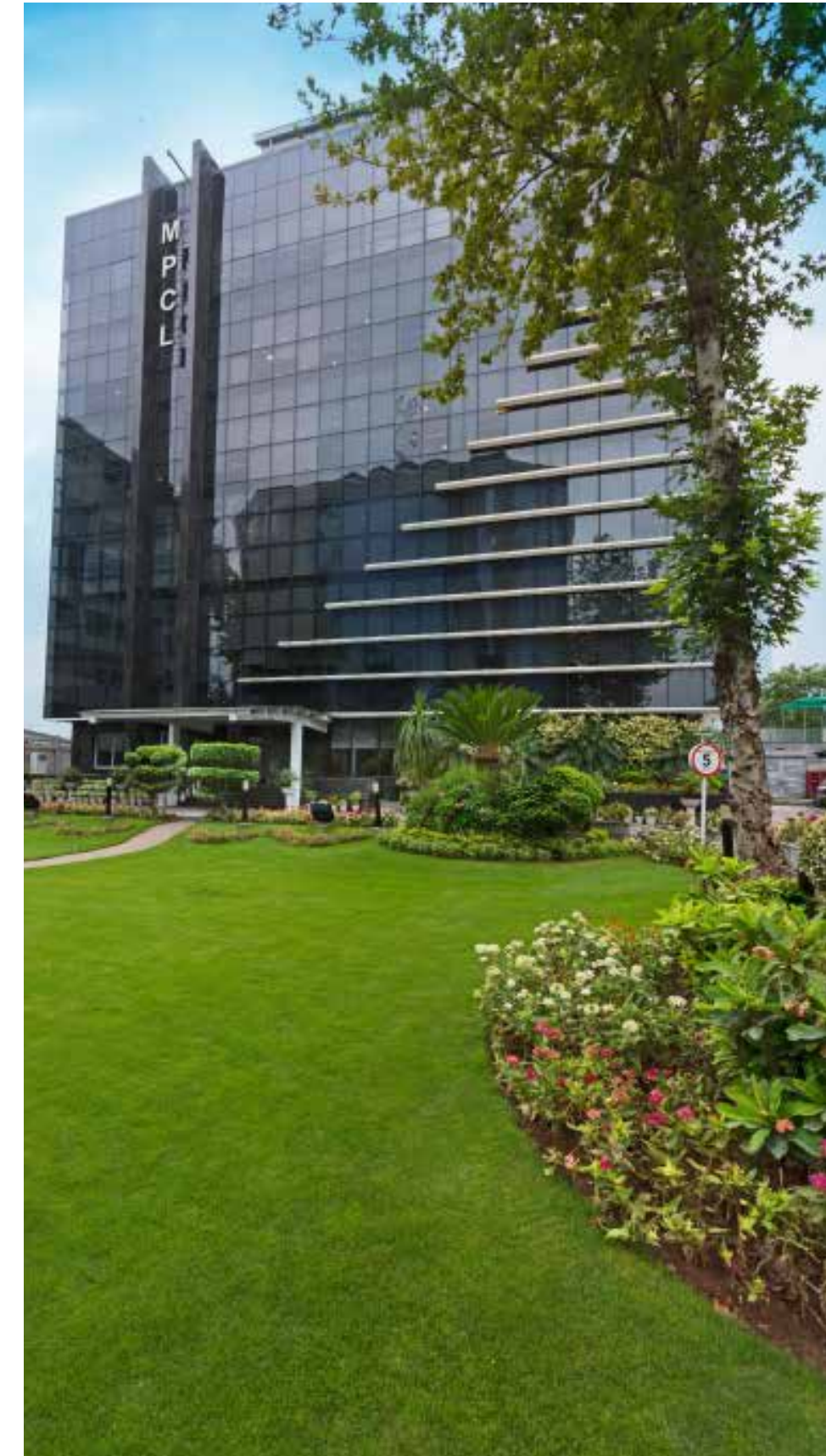
MPCL Head Office Building - Islamabad
