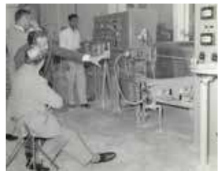
Aluminium Rod Extrusion Plant installed
