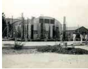
Pakistan Cables Factory SITE, Karachi
