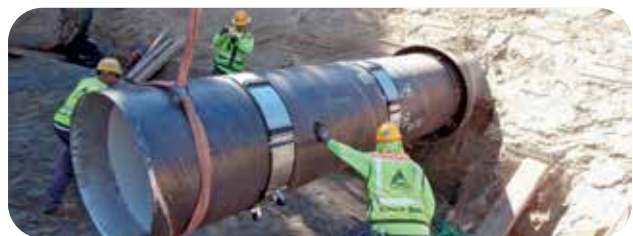
Steel line pipes are primarily used in transmission pipelines in the oil, gas, and water sectors. These line pipes are also used in construction, usually as piles at ports and jetties.
