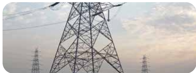
Secure reliable power sourced from CS Energy
