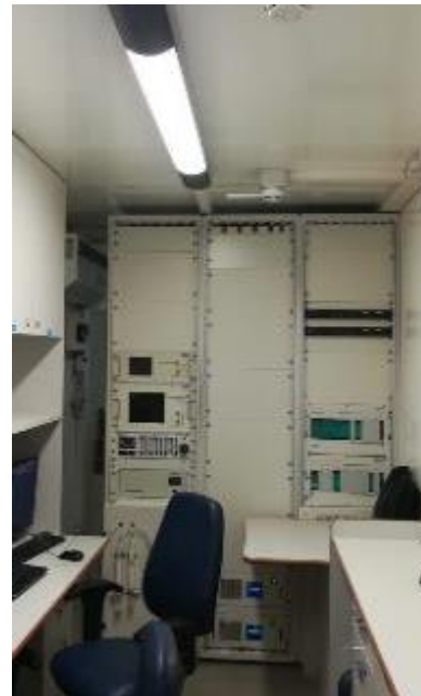
Mud Logging Unit
