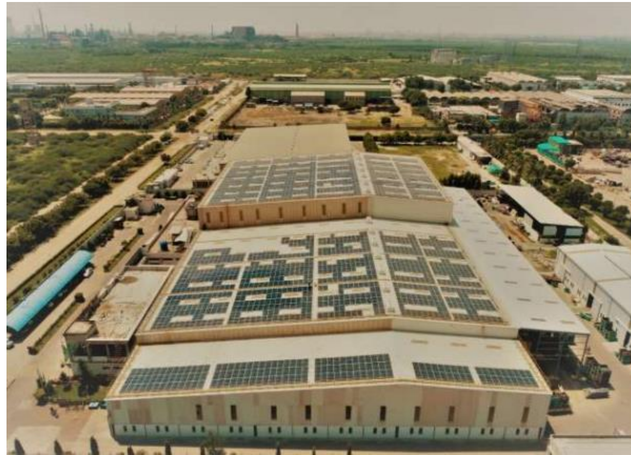
1 MW Solar Plant @ ASC
