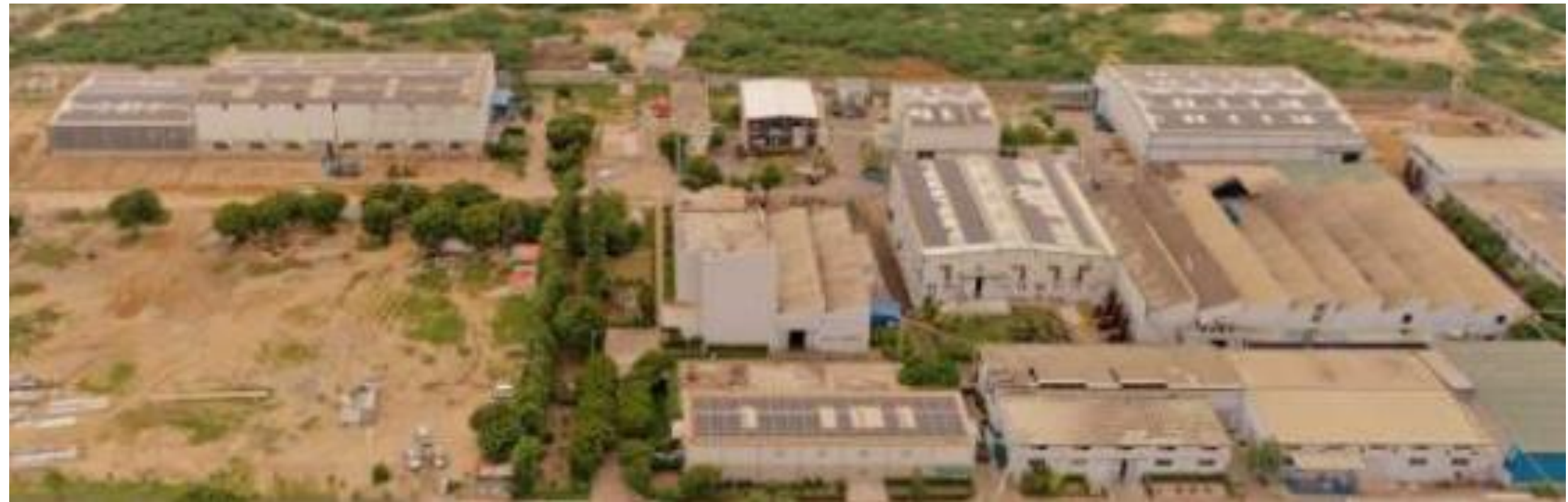
1 MW Solar Plant @ AIL
