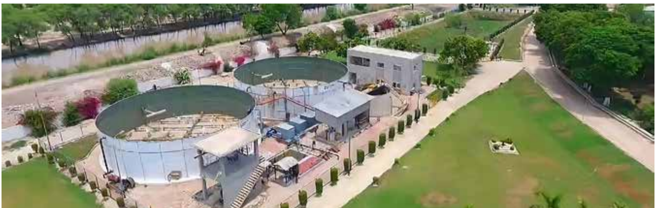
Effluent Treatment Plant
