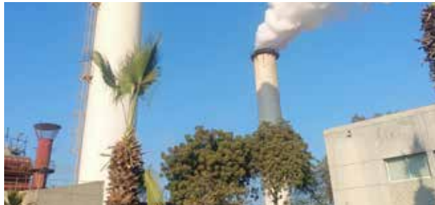
Fly Ash Recovery System
