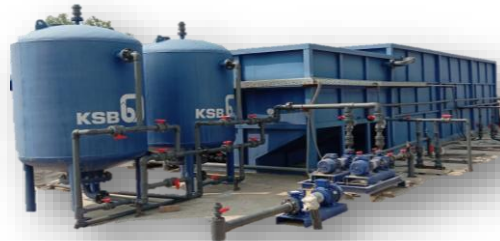
Sewage Treatment Plant
