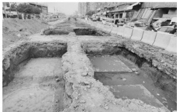
KARACHI: A view of slow work progress on Green Bus Project near Capri Cinema irks commuters.-INP
