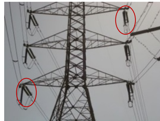
Typical Porcelain Application in Transmission Lines
