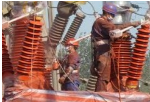
Typical substation insulators being coated
