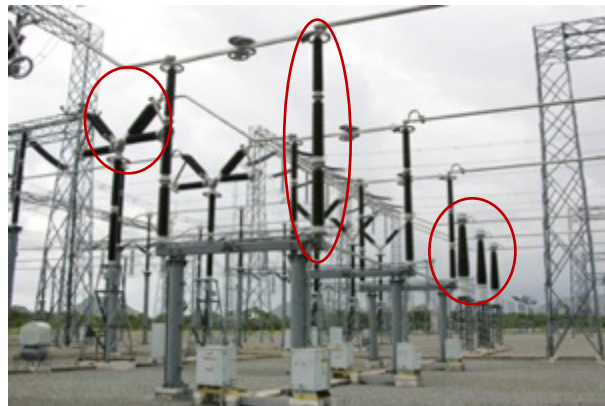
Typical Porcelain Application in Switchgear
