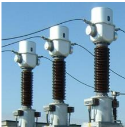
Typical Current Transformer Configuration
