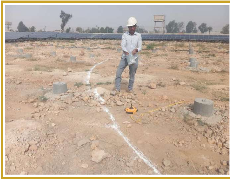
Site survey and turbine layout marking underway at the Noriabad site
