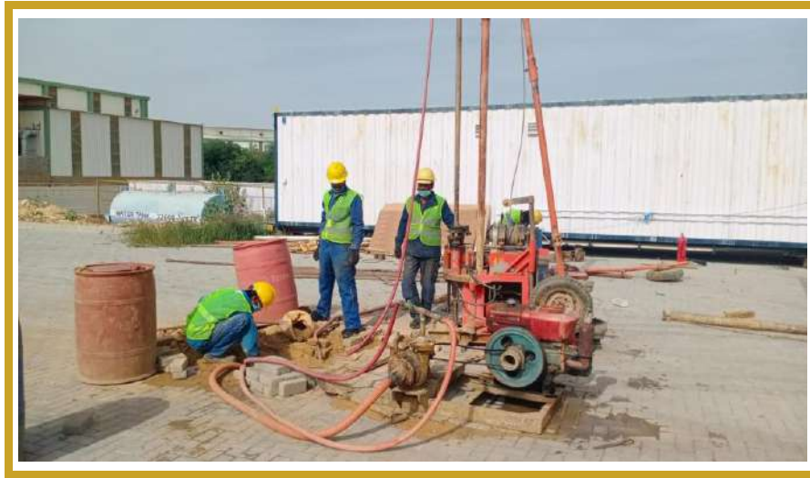
Soil investigation works in progress at the Noriabad site
