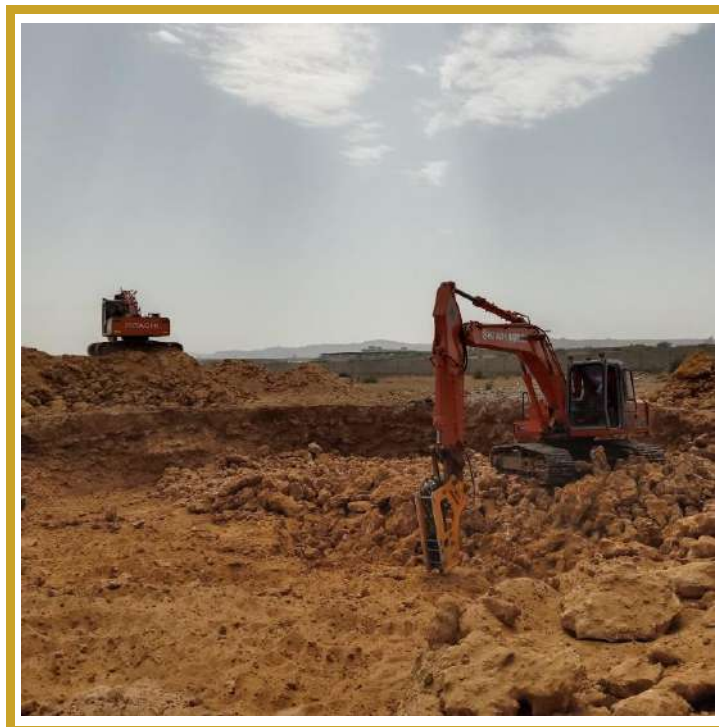
Foundation excavation works underway at the Noriabad site
