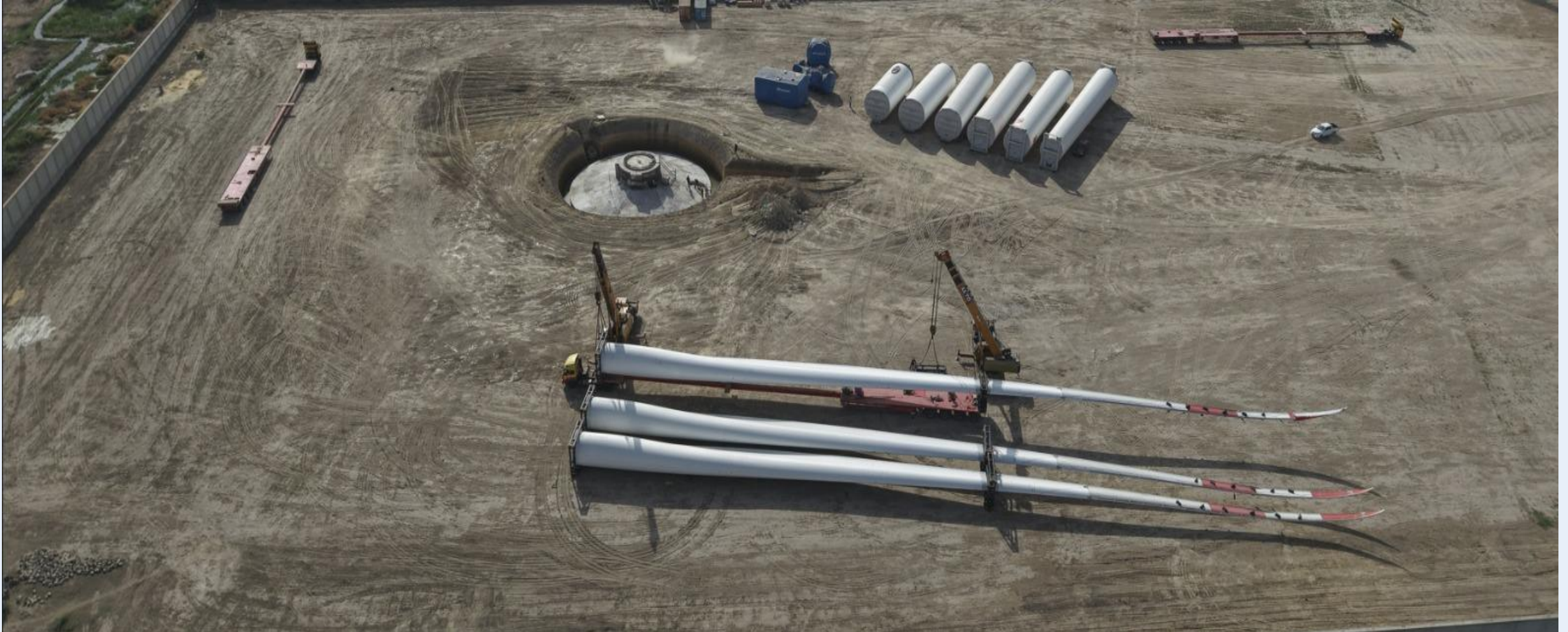
Turbine foundation and anchor cage, September 2026.
