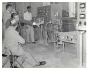
Aluminium Rod Extrusion Plant installed
