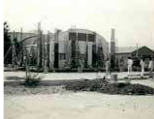
Pakistan Cables Factory SITE, Karachi
