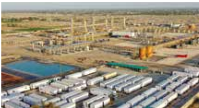
Sachal Gas Processing Complex, Mari Field, Daharki
