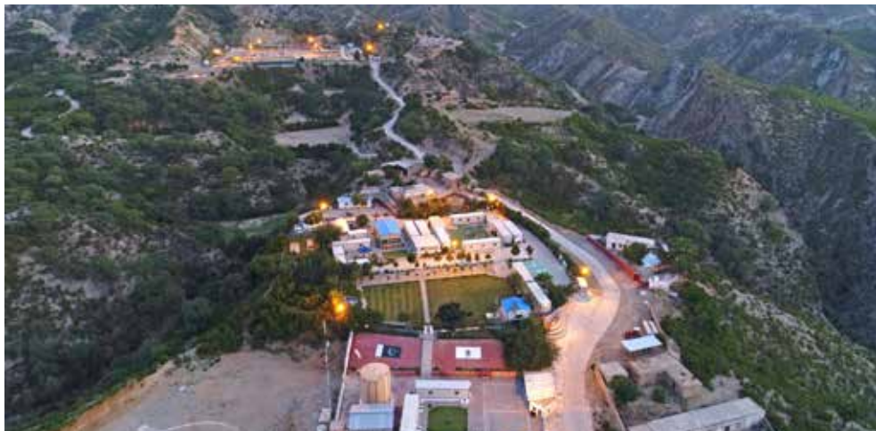
Halini Oil Field, Karak Block - Punjab Producing Wells 2, MPCL Working Interest 60%, JVP: MOL 40% Production - Gas: 1 MMSCFD, Oil: 700 BBLs per day
