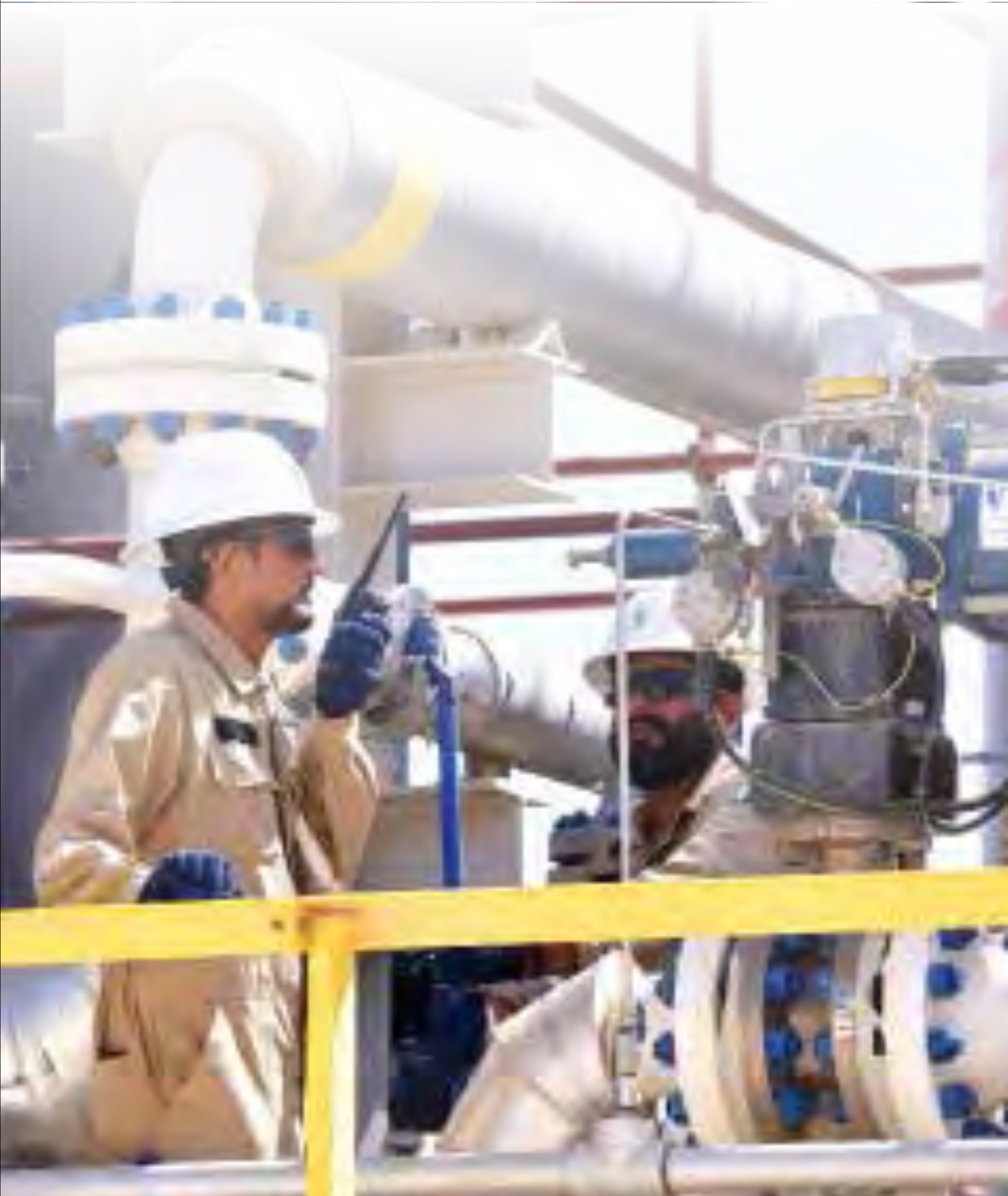
SGPC Plant, Mari Gas Field, Daharki - Sindh
