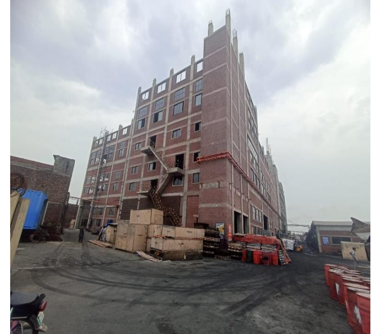
Building for Mixing Department PKR 388.0 Million
