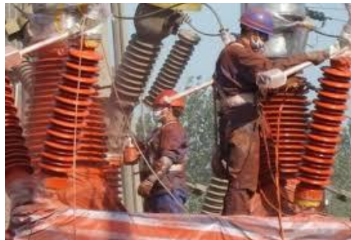
Typical substation insulators being coated
