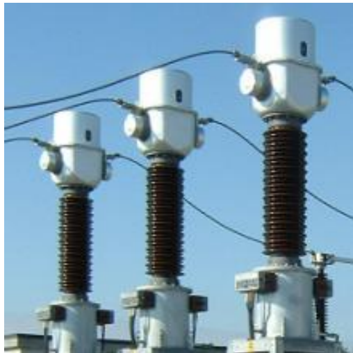
Typical Current Transformer Configuration
