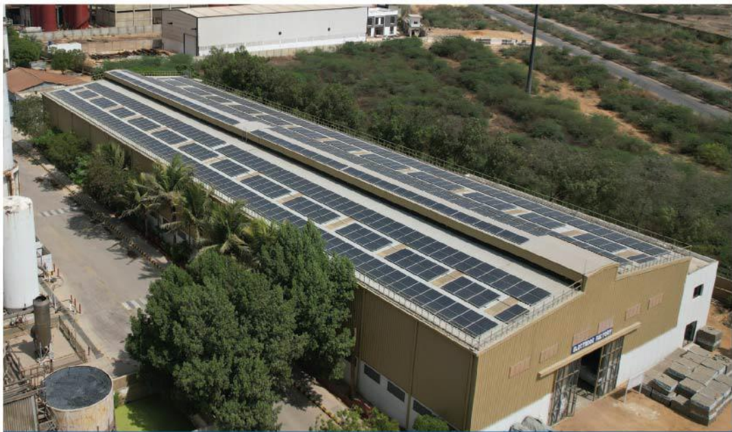
Electrode manufacturing plant at Port Qasim with 250 kWh solar energy.
