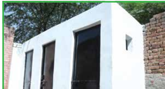
Washrooms installation in community schools
